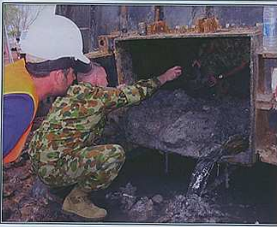
The Royal Australian Army bomb disposal crew removing small UXO from the obstruction strainer, watched by Aaron Bruce of Hall.
